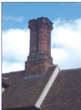
Chimney and roof in good repair
