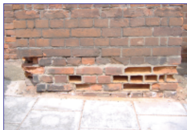
The effect of cement mortar on historic brickwork
