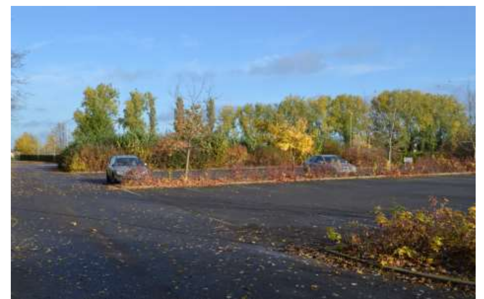
VIEW 7: Academy car park
