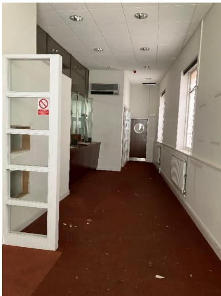
Part of the banking hall on the ground floor:
