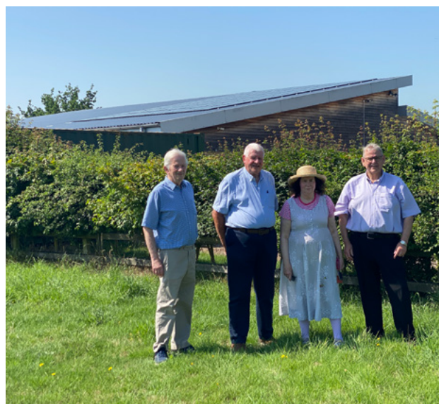
Solar installation at Honington & Sapiston Village Hall
