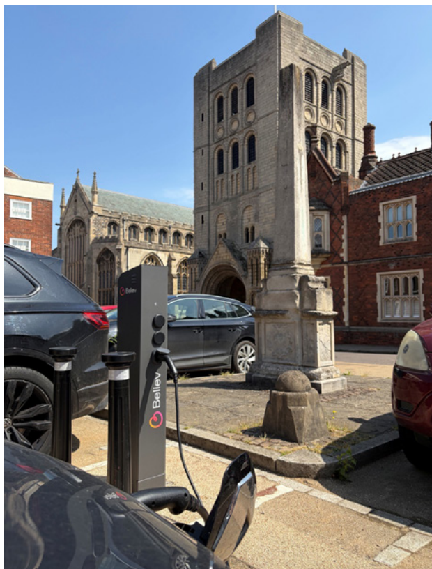
New EV chargers at Chequers Square, Bury St Edmunds
