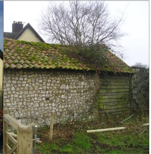
(fig 28 ) Pantiled roof, clunch block and timber-framed & weather boarded walls
