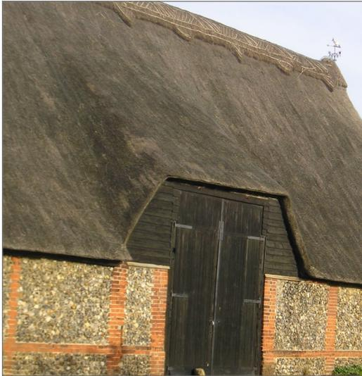
(fig 25) Water reed thatch, red brick banding & flint rubble
