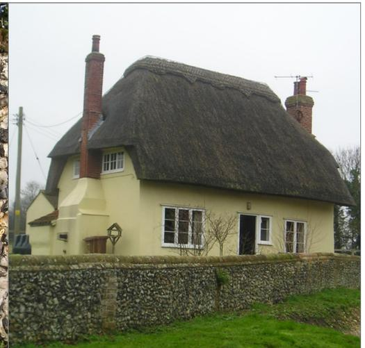
(fig 32 ) Rendered timber frame and long straw thatch at the Thatched Cottage, Lower Green
