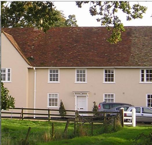
(fig 30 ) Plain tile roofs and rendered timber frame at Lodge Farm Lower Green
