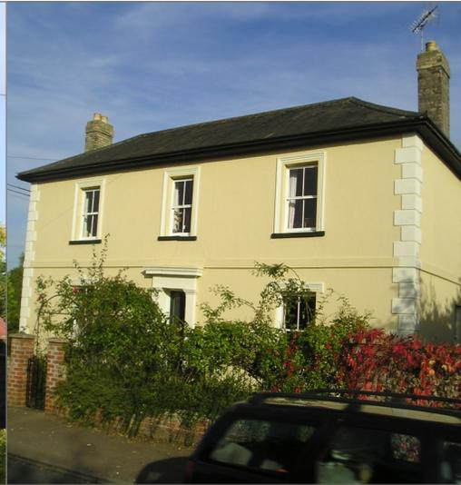
(fig 27 ) Stucco on brickwork, slate roofs and gault brick chimney stacks in Middle Green.
