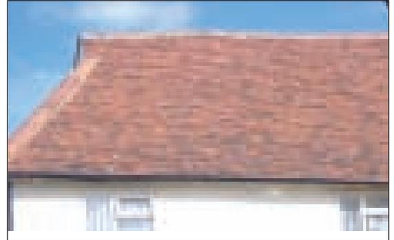
*Photo 26 (above): Example of clay plaintiled roof*
