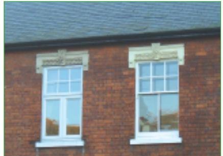
*Photos 9 and 10: comparisons of sash windows and uPVC replacements. Note how the frames of the uPVC windows are larger and flatter, they open differently and do not have the same three-dimensional appearance of the historic windows*
