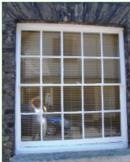
*Photo 5: small-paned sash window without horns*
