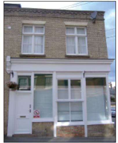
*Photo 17: former shop on Victoria Street with a parapet roof*
