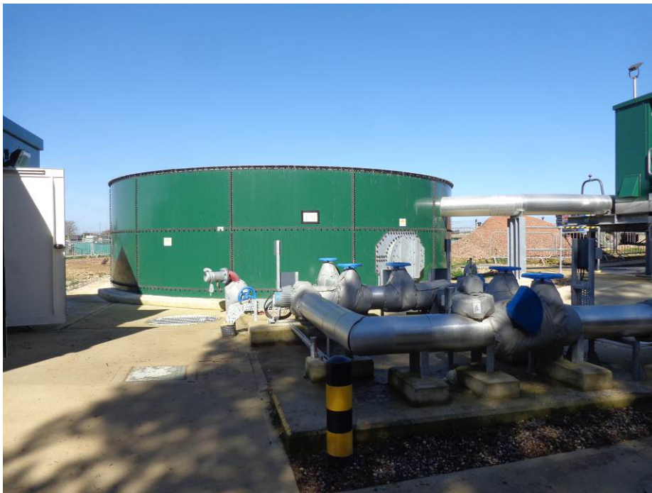
Photograph 1 Balance Tank
