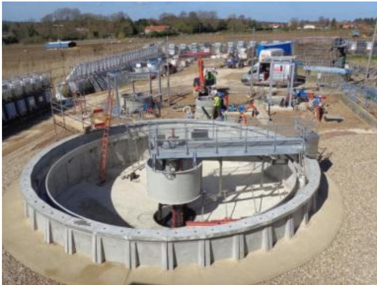
Photograph 6 New Final Settlement Tank
