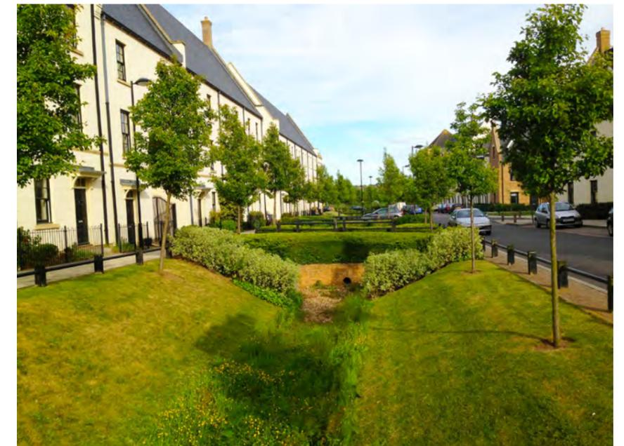
Figure 8 - Example of a method of Sustainable Urban Drainage
