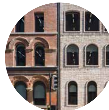
Fig.113 Responding to historical context through window sizes, shape and banding
