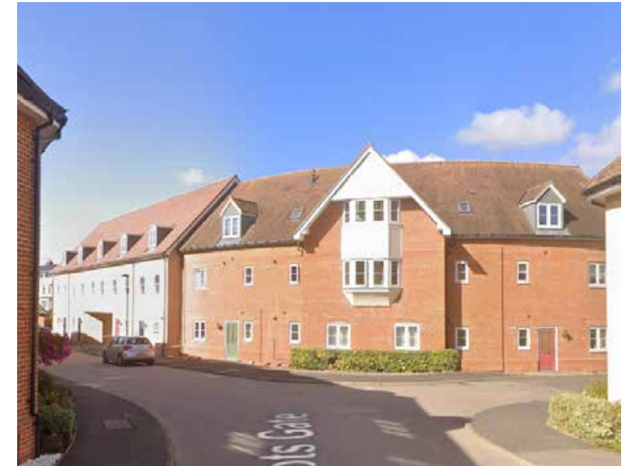
Fig.93 Example of marking key corners or junctions with a change in roof profile, Abbots Gate, Bury St Edmunds
