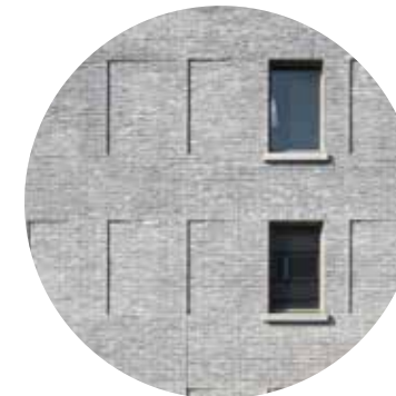
Fig.118 'Blind windows' for grid alignment
