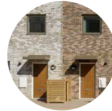
Fig.142 Paired front doors
