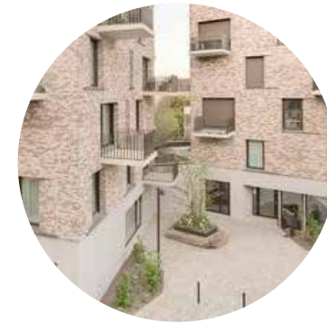
Fig.164 Base Expression, difference in brickwork, precast concrete for community hub.
