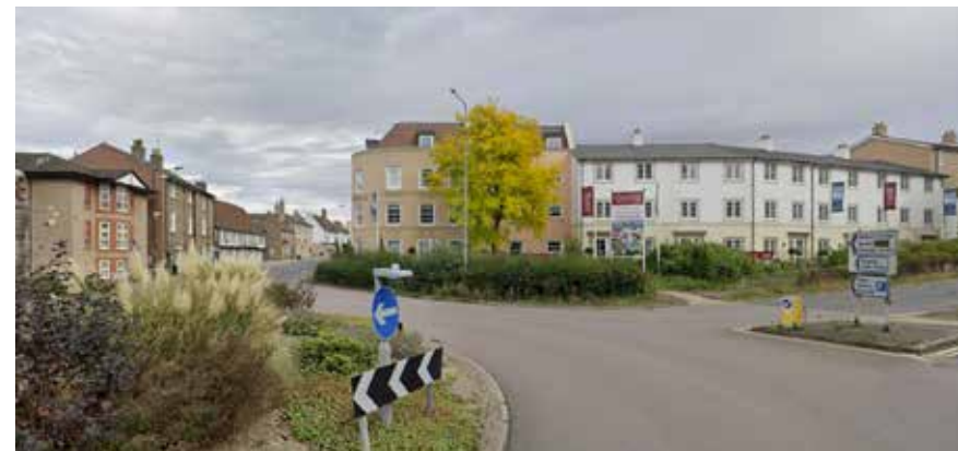
Fig.91 Stitching into existing context with a varied roof line and change in massing at Risbygate Street, Bury St Edmunds
