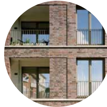
Fig.187 Top: Playful Stable Yard windows, bottom: Stable House Inset balconies, aligned windows
