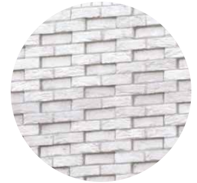
Fig.166 Expressed textured base adding interest at ground floor
