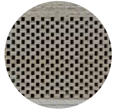
Fig.167 Expressed textured base adding interest at ground floor
