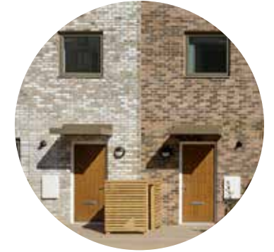
Fig.120 Paired front doors
