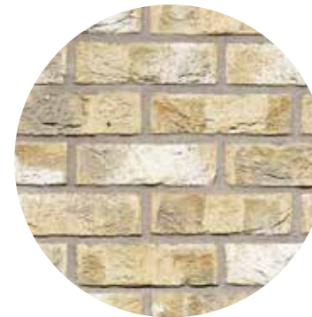
Fig.158 Ground floors light buff brick
