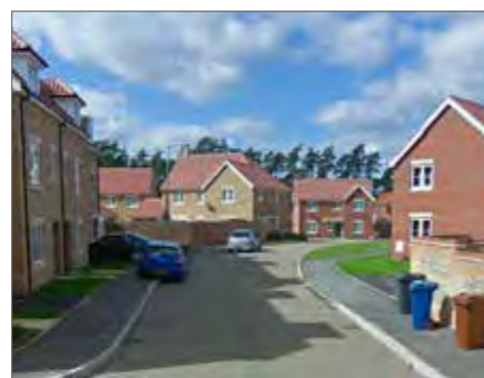
Evergreen Way - 29 dph Detached, semi detached and terraced housing, some 3 storey, minimum or no front gardens
