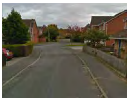
Miles Hawk Way - 18 dph Detached houses large plots, small front gardens, green spaces
