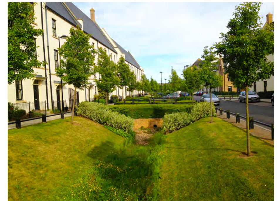
Figure 5 - Example of a method of Sustainable Urban Drainage Image from https://pipedup.files.wordpress.com/2013/06/upton-edit.jpg
