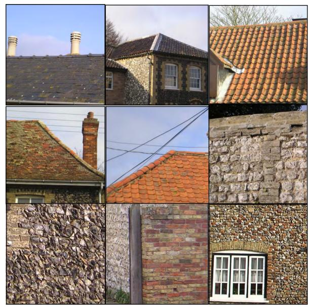
Top left to bottom right: Welsh slate, black glazed pantiles; red clay pantiles; local mixture of gault clay and red hand made plain tiles; flat-profile imported clay pantile; chalk block and gault brick; napped flint with gault brick dressings; local red and gault brick mix: and brick and flint rubble wall with segmental arched gault brick lintel.
