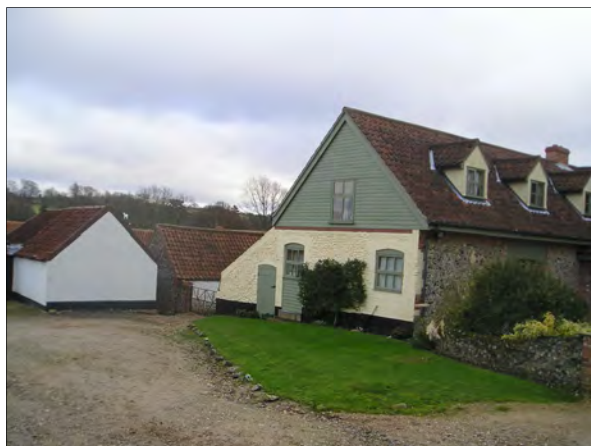
(Fig 37) French Hall Farmhouse, converted from a barn and cart shed retaining original external walls and roofs
