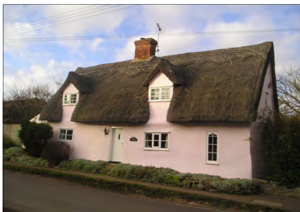
(Fig 24 ) No 7 Bridge Street, a 17th-century timber-framed, rendered and thatched cottage
