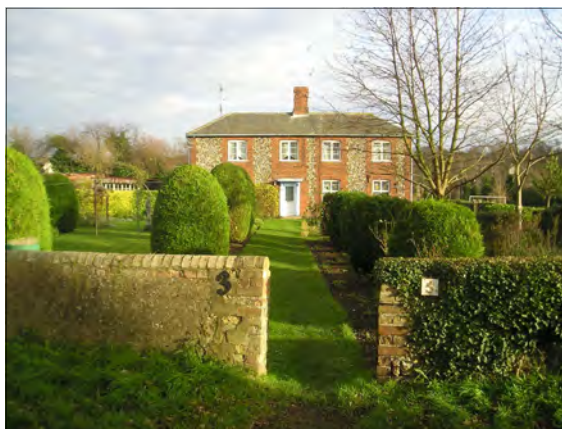
(Fig 30 ) No 3-5 The Street, in the prevailing 19th-century form with flint and brick walls, square plan & hipped slate roof
