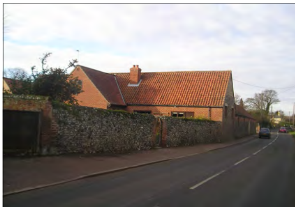
(Fig 35) The Barn, French Hall, a farm building reconstructed for residential use retaining the old Farmstead boundary wall
