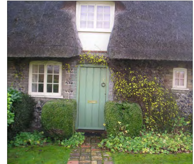
(Fig 51) Traditional painted timber casement windows and simple boarded door.
