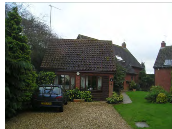
(Fig 58) The buildings in Park Close make a neutral contribution to the character of the conservation area
