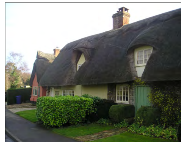
(Fig 40 ) A fine group of straw thatched cottages with eyebrow dormers in Church Road
