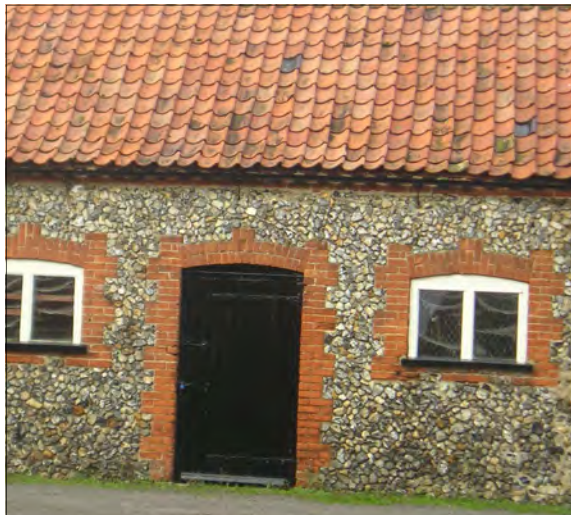
(Fig 50) Red clay pantiles, brick corbel eaves course, flint rubble walls with red brick quoins and segmental brick arches
