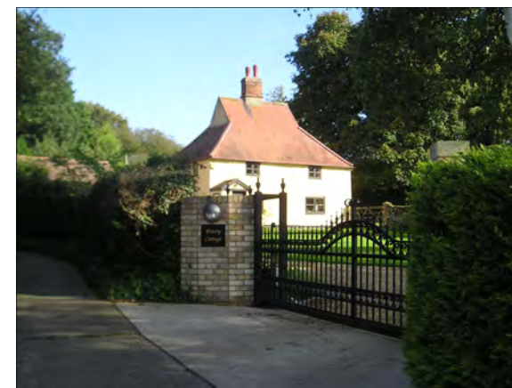
(Fig 20) Priory Cottage
