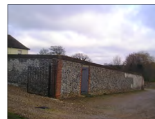
(Fig 43 ) Flint rubble boundary walls
