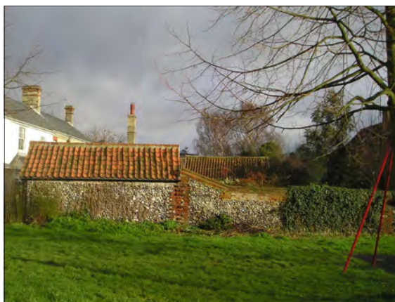
(Fig 29 ) Surviving walls probably from the former Trinity Farm in Bridge Road
