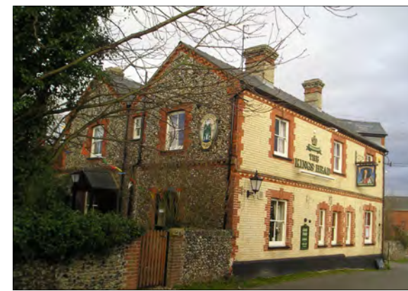
(Fig 25) The Kings Head built in polychrome brickwork and traditional flint and brick.
