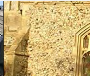
(Fig 49) Flint rubble with limestone dressings
