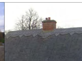
(Fig 45 ) Sedge Ridges in water reed thatch.
