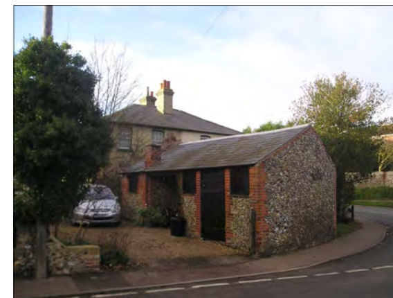
(Fig 31 ) 2 & 4 Newmarket Road, a square plan 19th-century plan houses with a neat flint stable in its forecourt
