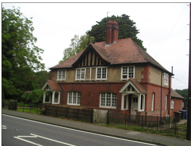
(Fig 12) London Road Estate Cottages
