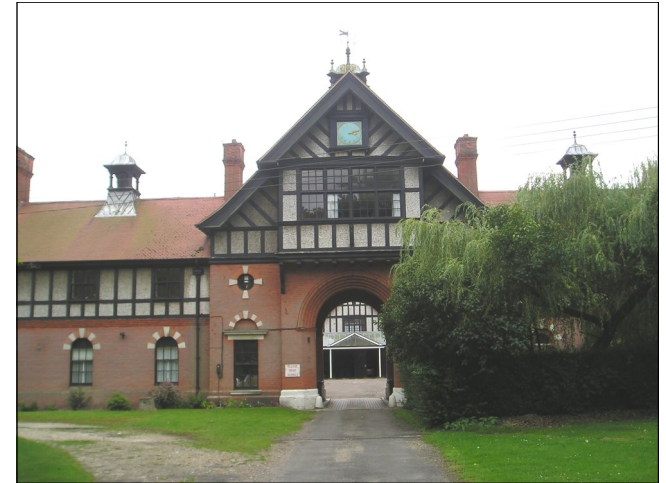
(Fig 30) North Entrance to Hall Stables
