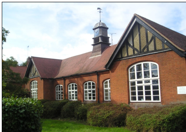
(Fig 56) Elveden VA Primary School
