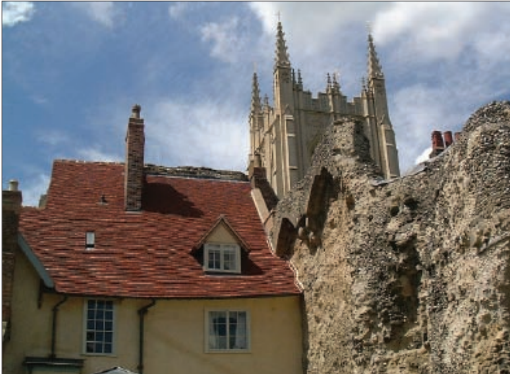
Photo 58: Rear roof slope of the West Front
