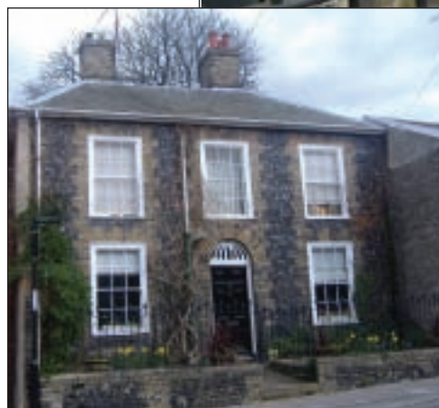
Photo 60: Building details found in the Brackland area
