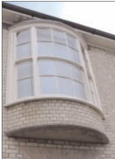
Photo 36: First floor bay of 90 Risbygate Street
