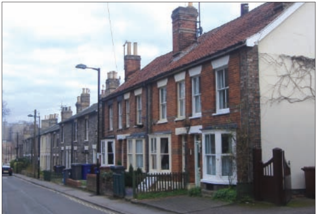
Photo 59: Typical properties in the Brackland area.
