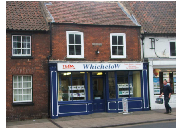
C19 th house with early C20 th shop front High Street
