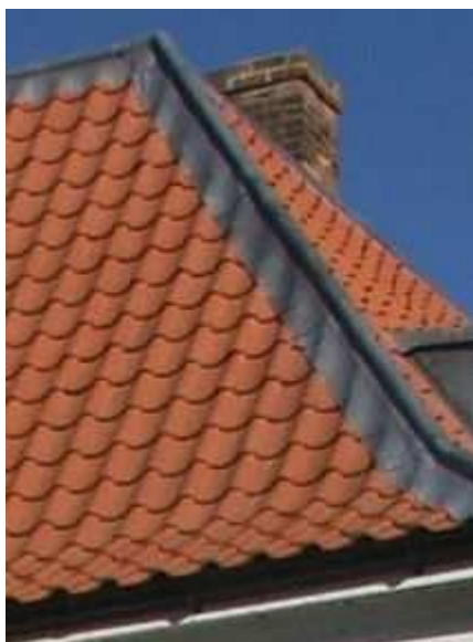
Roof detail Riverside Lodge High Street
