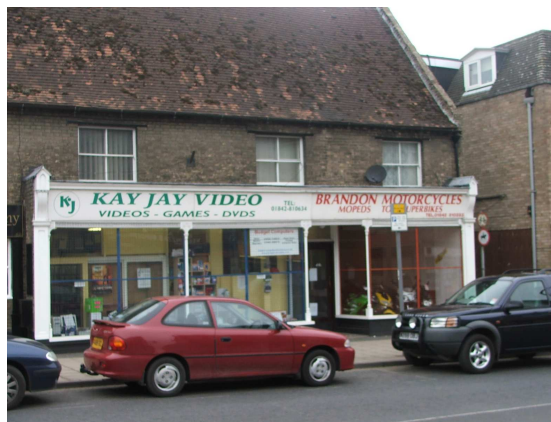
Early C29th shop front inserted into C16th house 49/51 High Street
