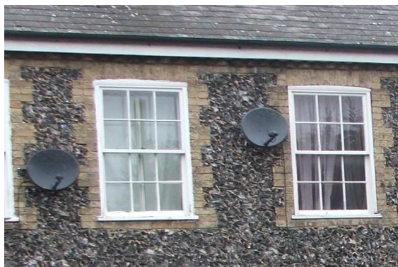
Upvc windows, satellite dish on C19th house in London Road
