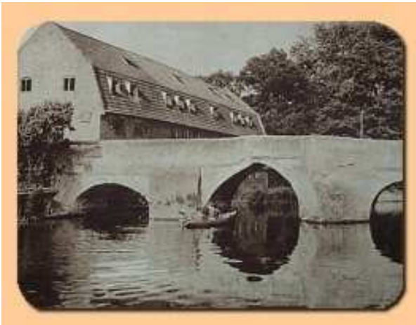
The old stone bridge across the little Ouse
