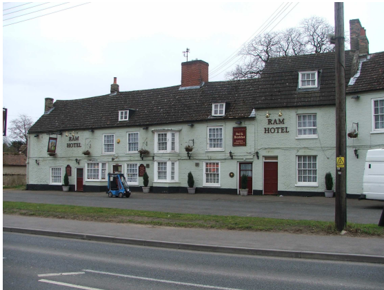
C 16 th timber framed Ram Inn Bridge Street
