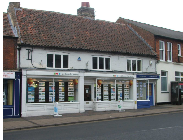
C16th timber frame house with early C20th shop front 16-22 High Street
