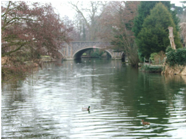
View of the bridge at north end of High Street
