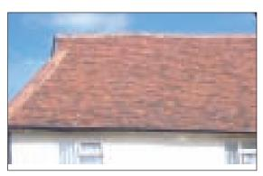
Photo 26 (above): Example of clay plaintiled roof Photo 27 (left): Patterned slates on the Community Centre roof
