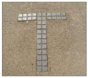
Photo 75: Rolled gravel with blue clay setts in Market Hill
