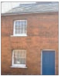
Photo 44: Example of rat-trap bond on properties in Station Road
