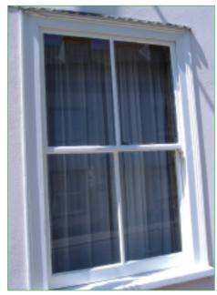
Photo 6: large-paned sash window with moulded horns on the top sash
