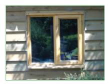
Photo 8: storm-proofed casement. Note how the glazed area of the left-hand fixed light is larger than the right-hand opening light and how the opening light stands proud of the frame
