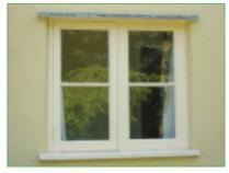
Photo 7: flush-fitting casement. Note how the right-hand fixed light is the same size as the left-hand opening light
