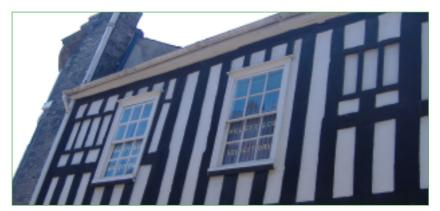
Photo 4: 16th century blocked mullion windows with inserted sash windows between. Note the different sizes and proportions of the windows
