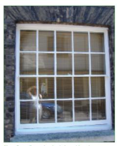
Photo 5: small-paned sash window without horns
