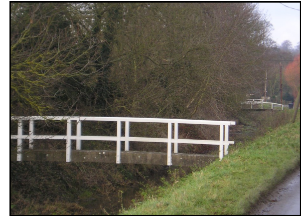
The foot bridges across the Kennet in The Street
