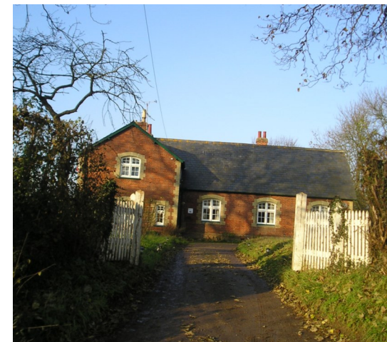
The former national school, , Denham Road
