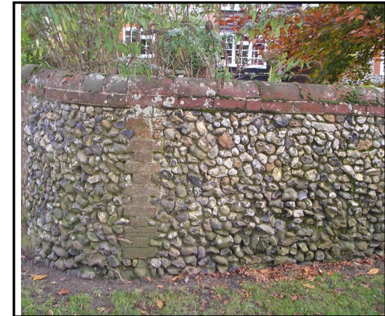
Flint Rubble & Brick Wall, Beechbrook House
