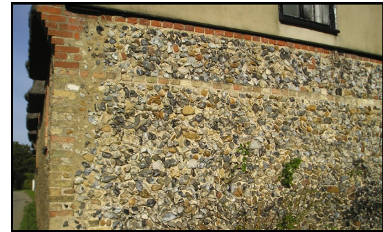
Brick, flint rubble & render
