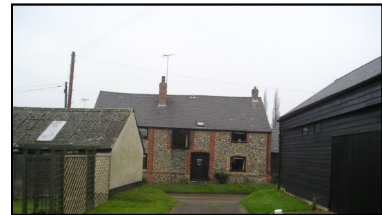
Slate, weatherboards red brick and flint rubble
