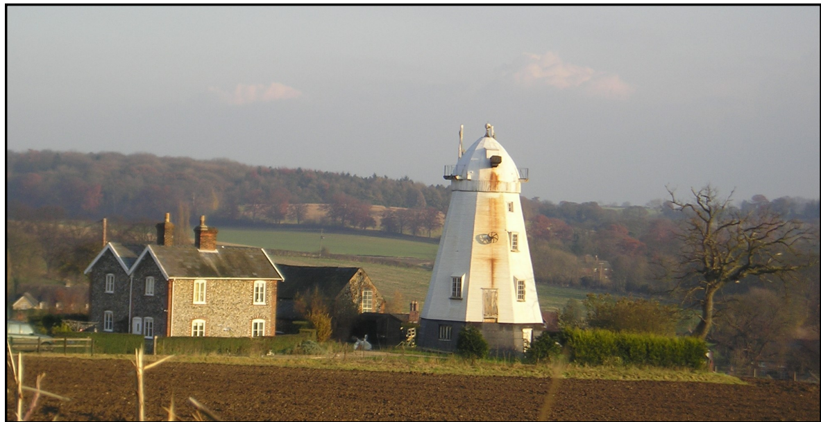
Lower Mill, Stores Road , an important group of buildings and a landmark visible from a wide area.
