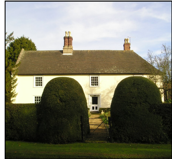
The Old Manor, formerly Hall Farm House is at the centre of an important group,
