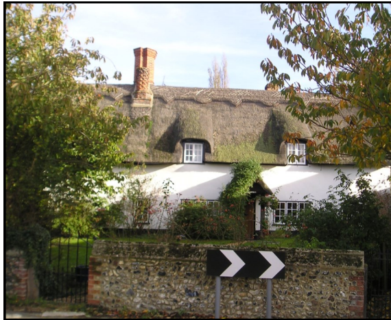
Flint garden wall of Ford Cottage, The Street
