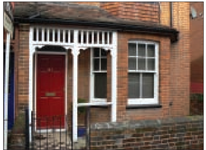
Photo 31: Open porches with decorated timberwork
