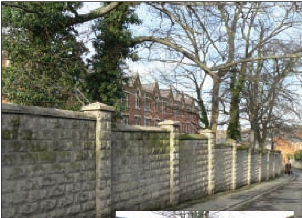
Photo 23: High blockwork walls partially obscure factory
