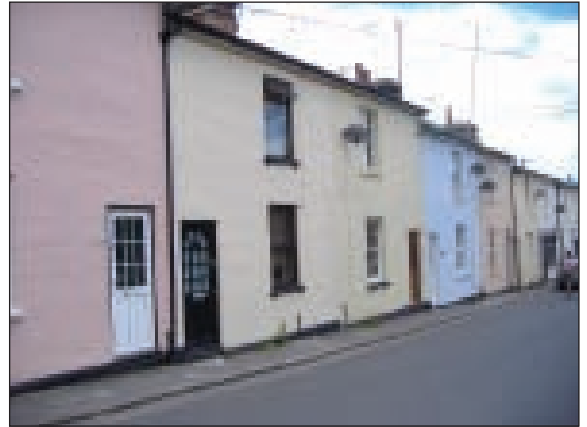
Photo 25: Mill Road, North
