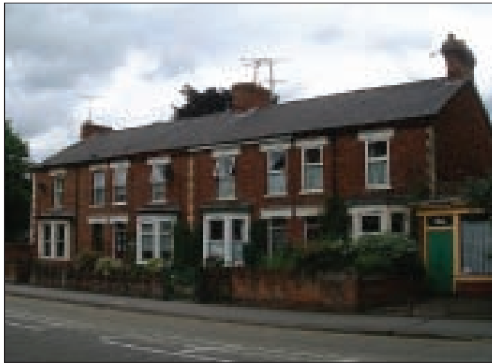
Photo 8: Terraces on Withersfield Road
