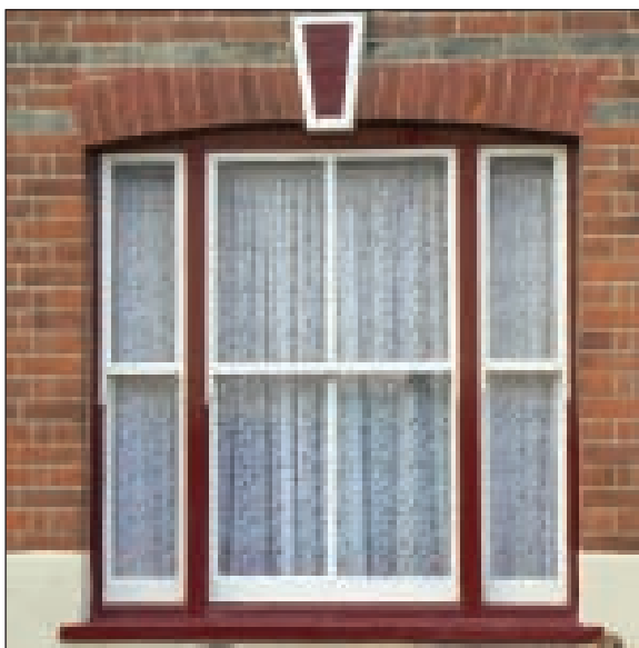
Photo 35: cambered brick arches over tripartite windows
