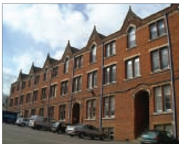
Photo 22: Factory Building built in French Gothic style
