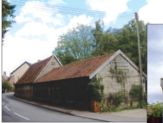
Photo 22: farm buildings in Bury Road
