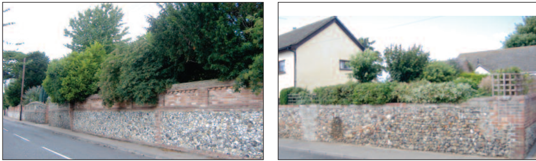
Photo 33: examples of flint walls
