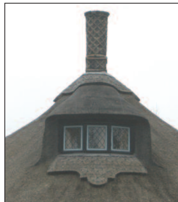
Photo 42: chimney and dormer of the Round House
