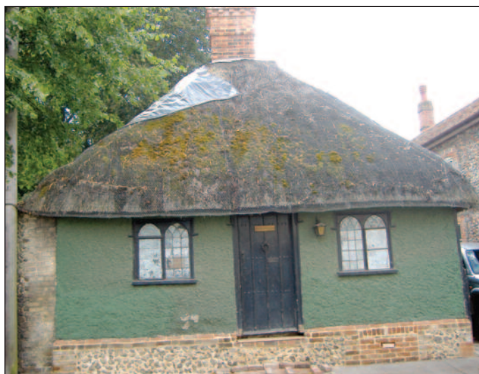
Photo 27: Early 19th century former lodge to Stayer Cottage
