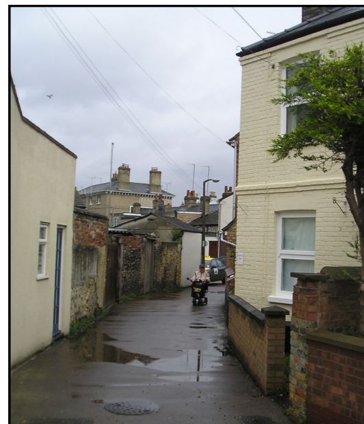
New Cut looking North
