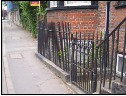
Railings, High Street
