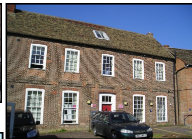
Cambridgeshire clay plain tiles and local red brick with lime mortar
