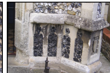
Knapped flint & limestone flushwork
