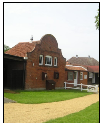
Kitchen Wall Box
