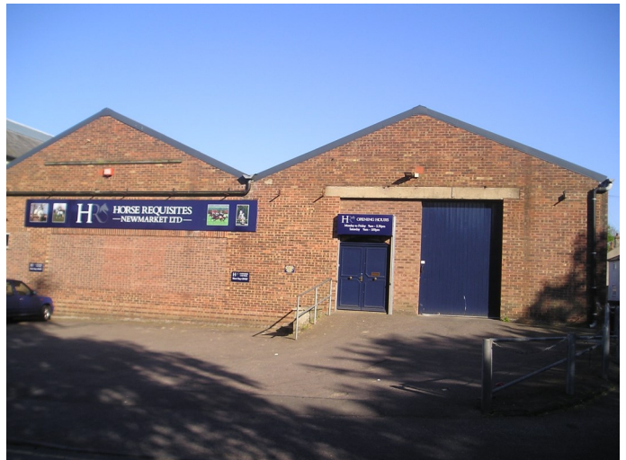
Visual intrusion – retail warehouse, Bear Lane, Fitzroy Street
