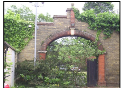
C18th entrance to Avenue Stables
