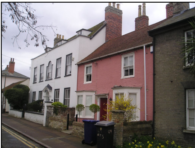
Boyce House & Havelock House
