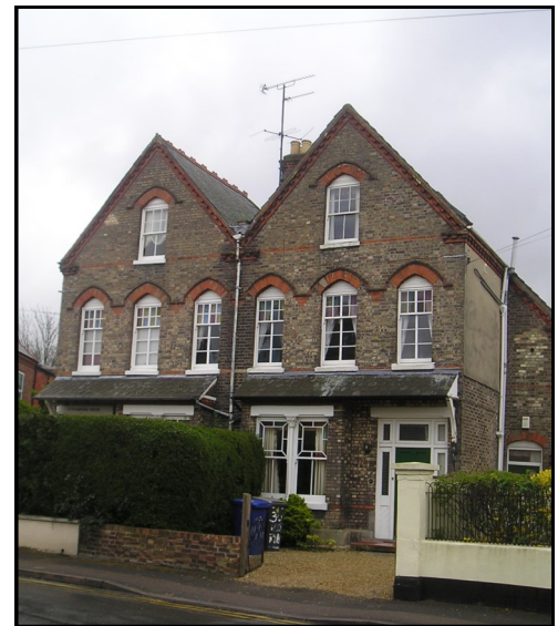
Denson Terrace: large, well detailed, semi-detached houses of the Edwardian period.
