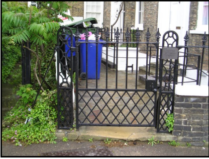
Railings, St Mary's Square
