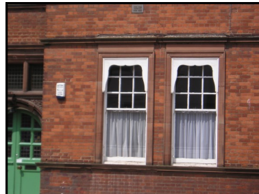
Edwardian sash windows & blind boxes
