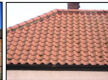
Red clay pantiles and painted cement render
