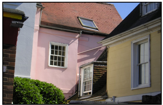
Georgian & Victorian sash windows
