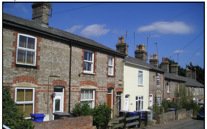
Replacement and traditional widows in adjoining houses.
