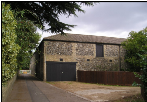
Hunworth House Stables
