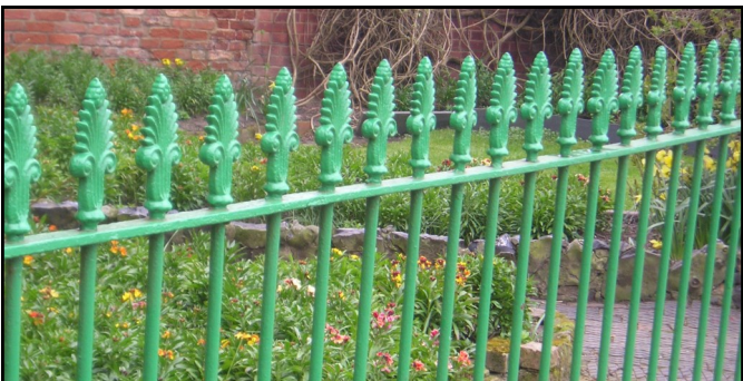
Railings of Osborne House
