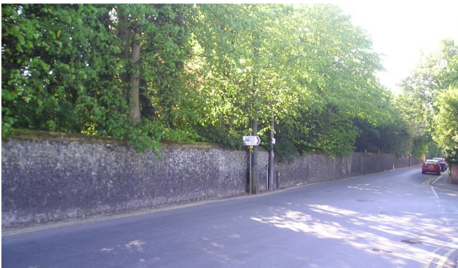
Boundary wall of Fitzroy Stables
