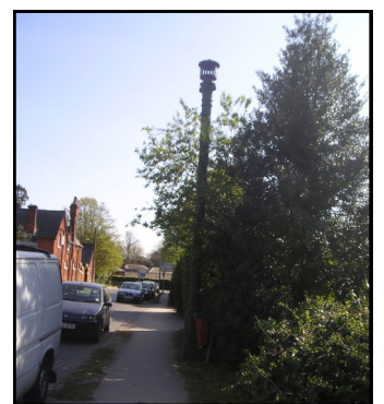
Old cast iron sewer vent
