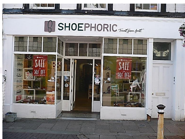
Examples of shop fronts incorporating the basic elements of good shopfront design and quality materials
