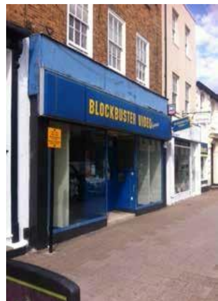
A badly designed shopfront with a poorly placed projecting box fascia
