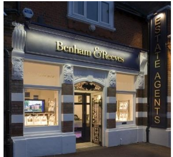
Cornice incorporating recessed lighting
