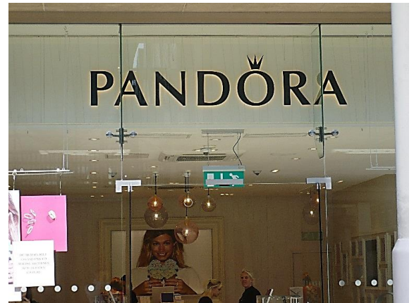
Example of halo style lighting
