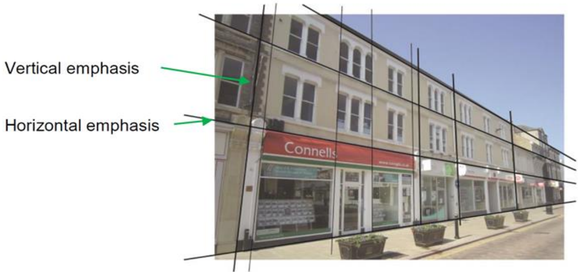
New shopfronts sympathetic to historic buildings
