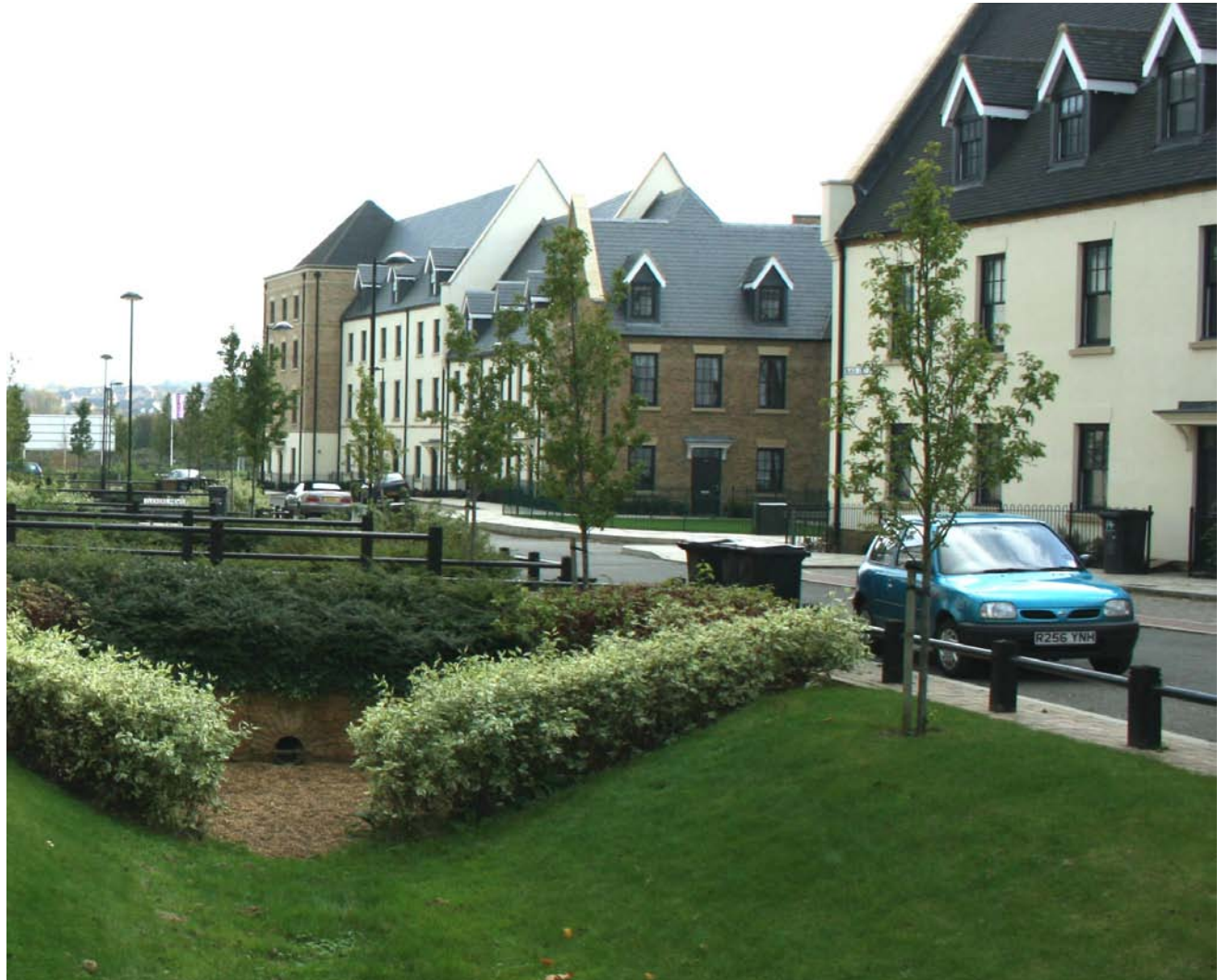
Example of swales forming an integral part of the overall design
