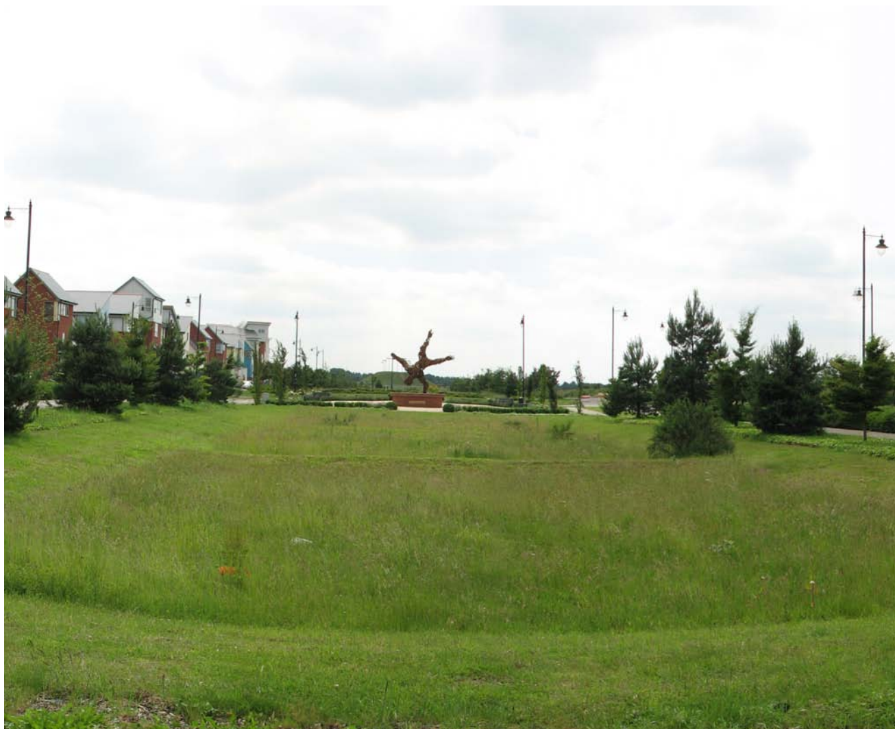
Infiltration basins forming a usable part of the open space
