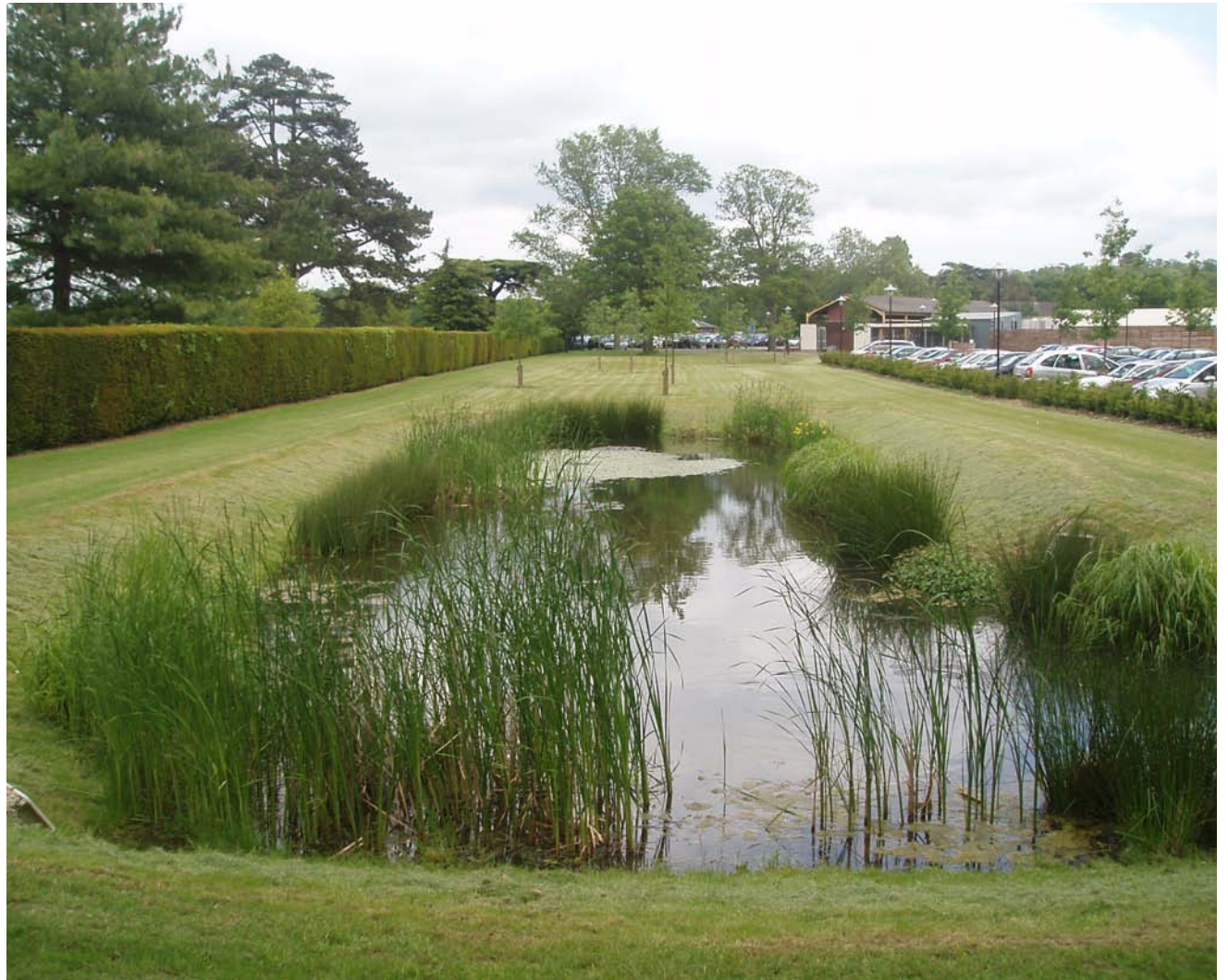
Combined infiltration basin with pond forming an attractive feature within the landscape structure.
