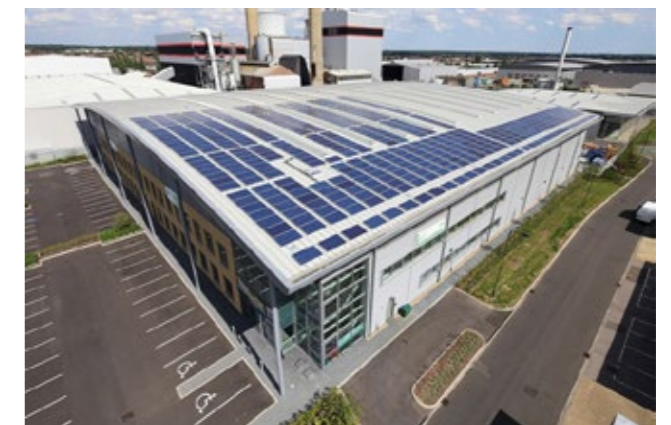
Fig. 39: Photo voltaic panels located on roof
