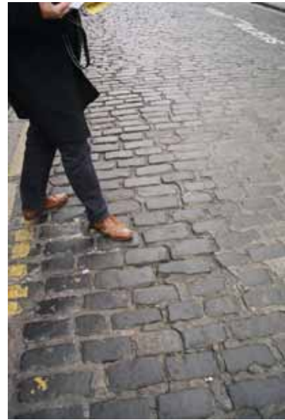
6.1 A variety of materials to be use in Highways
