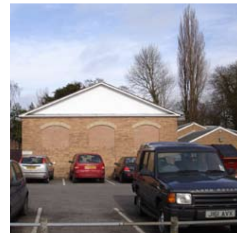
Figure 24 View of building group from car park
