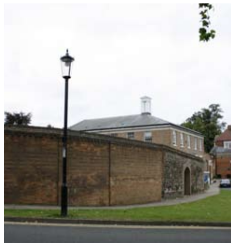
Figure 14 The wall to the Weymed site - partly brick and partly flint
