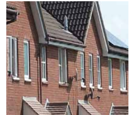
Red brick wall
