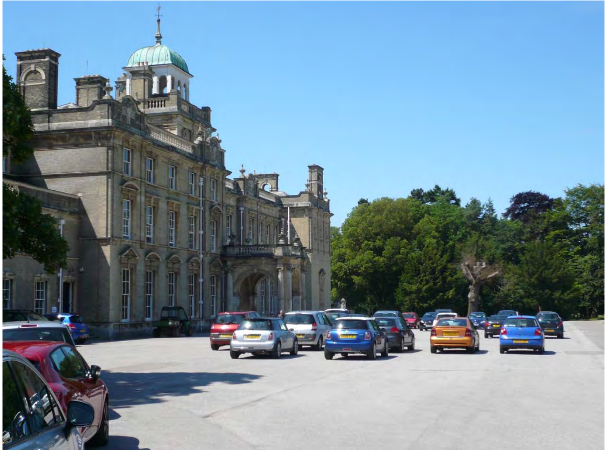
17: Car parking against the north front of Culford Hall. The school is committed to reducing car parking in front of the hall and returning the original parkland setting. See paragraph R.8.7.1.
