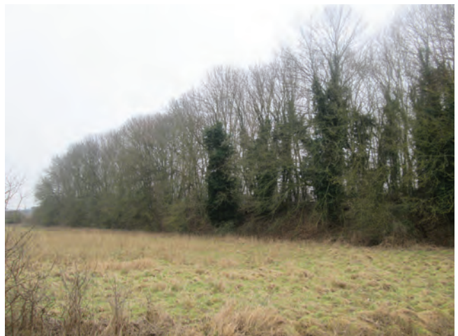
Part of the remaining length of railway embankment
