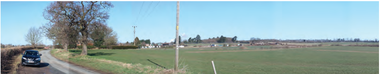
View from Rushbrooke Lane looking north towards A14 showing 33kV overhead power line
