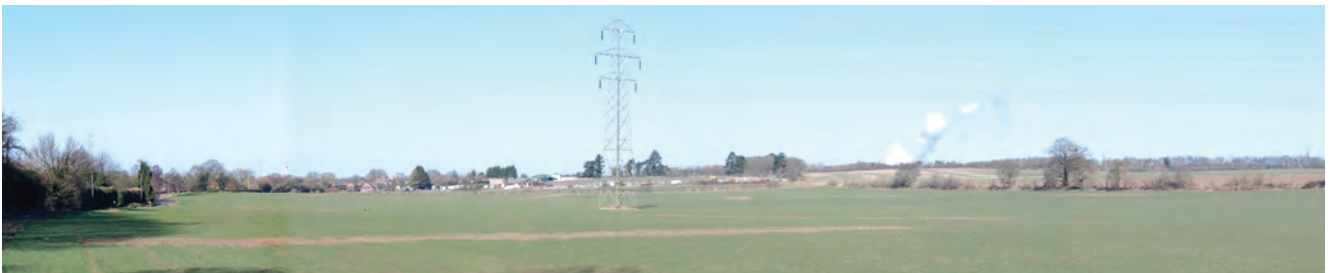
View north from public footpath near Rushbrooke Lane showing 132kV overhead power line
