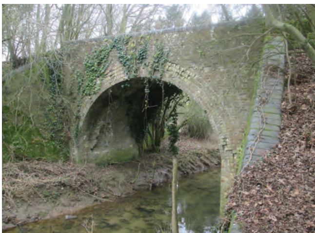
Former railway bridge over the River Lark
