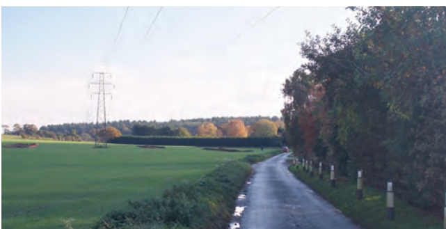
View south where 132kV overhead line crosses Rushbrooke Lane
