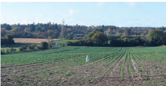
Typical distant view of 132kV overhead line looking west
