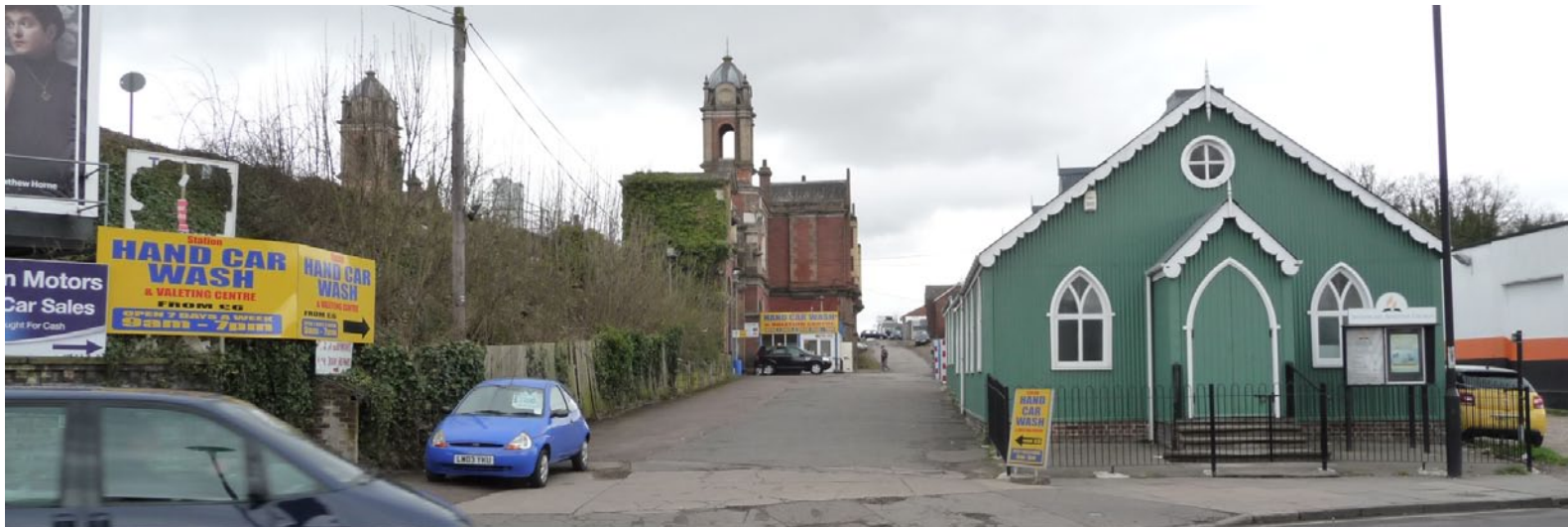
View of the rear of the station from Fornham Road
