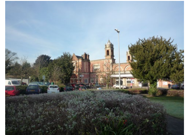
Station access road off Station Hill
