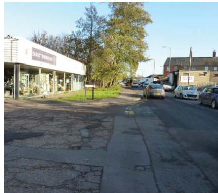
Vehicle entrance from Tayfen Road
