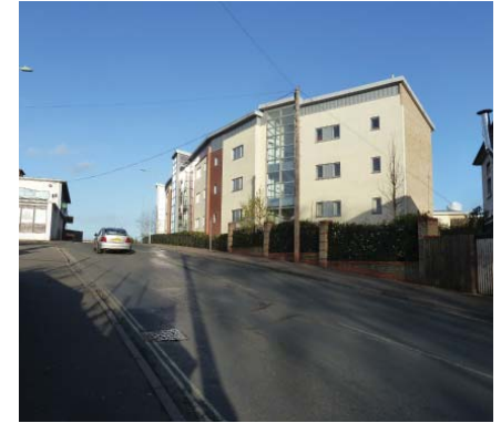
View along Station Hill
