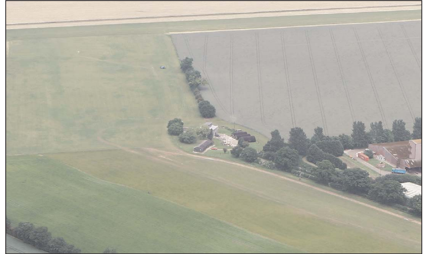
Aerial view of Control Tower and associated buildings
