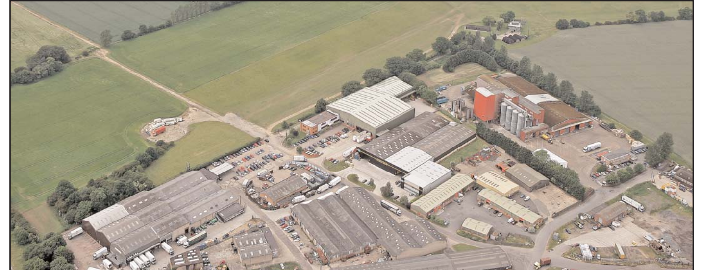
Aerial view of existing Rougham Industrial Estate and Airfield Control Tower
