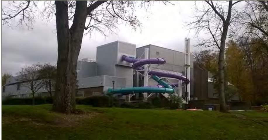
Figure 6: Photograph of Abbeycroft Leisure Centre taken during Ramboll Site Visit
