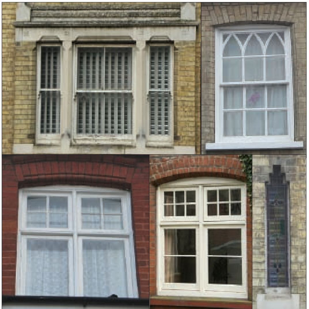
Photo 23: Windows range from sashes to casements
