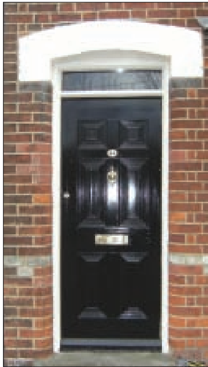
Photo 13: Fanlights over door openings provide additional light
