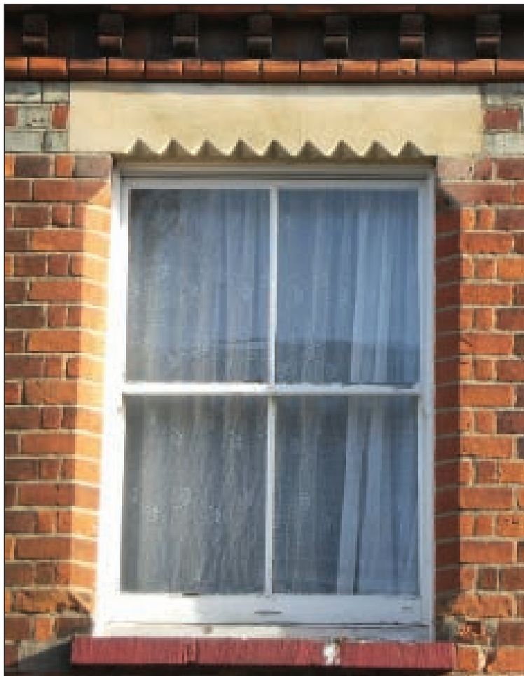
Photo 11: saw-toothed lintels and chamfered brick reveals decorate window openings
